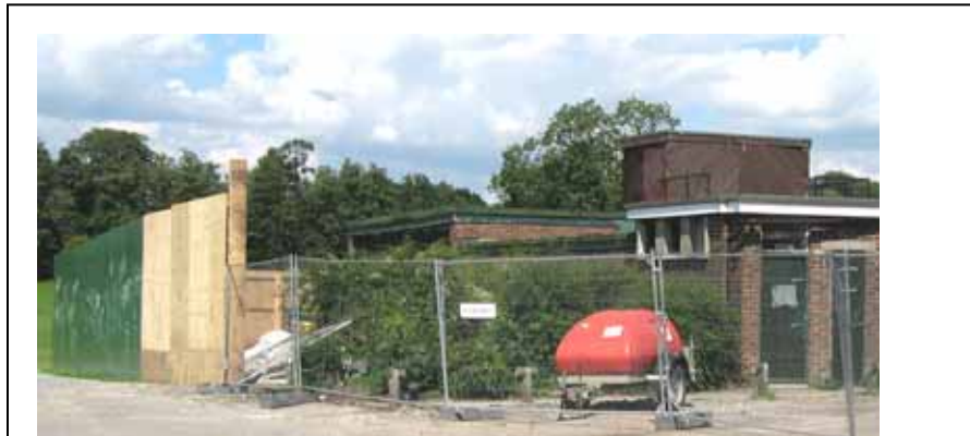
Final view of the old club house before it is demolished.
